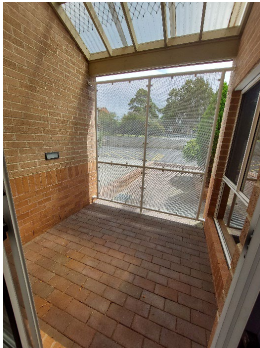
Image 14: Enclosed smoking area that doubles as an exercise yard
